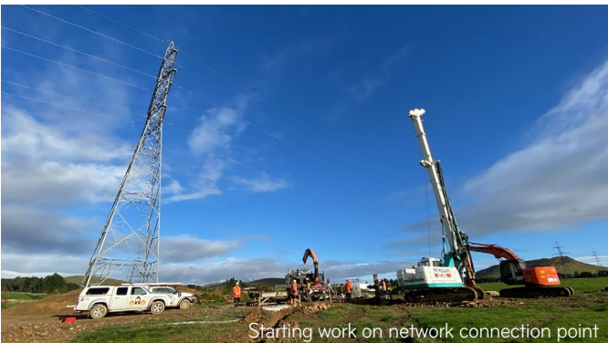
Starting work on network connection point
