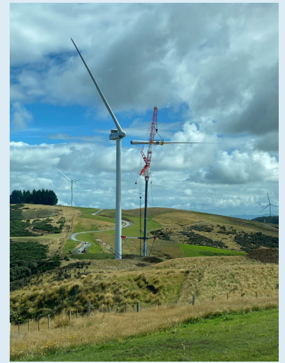
The biggest cranes you ever saw are used to assemble the turbines
