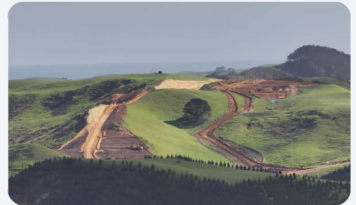
BULK EARTHWORKS ARE NEARLY COMPLETE
