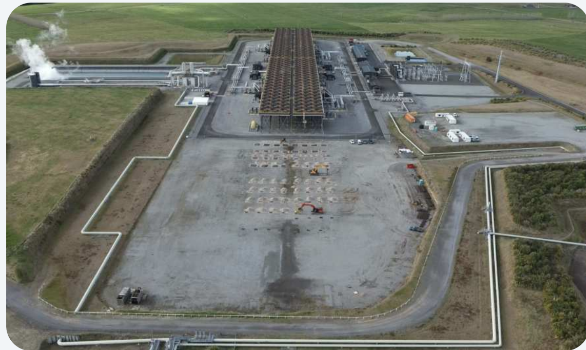
CONSTRUCTION START – MAY 2024
