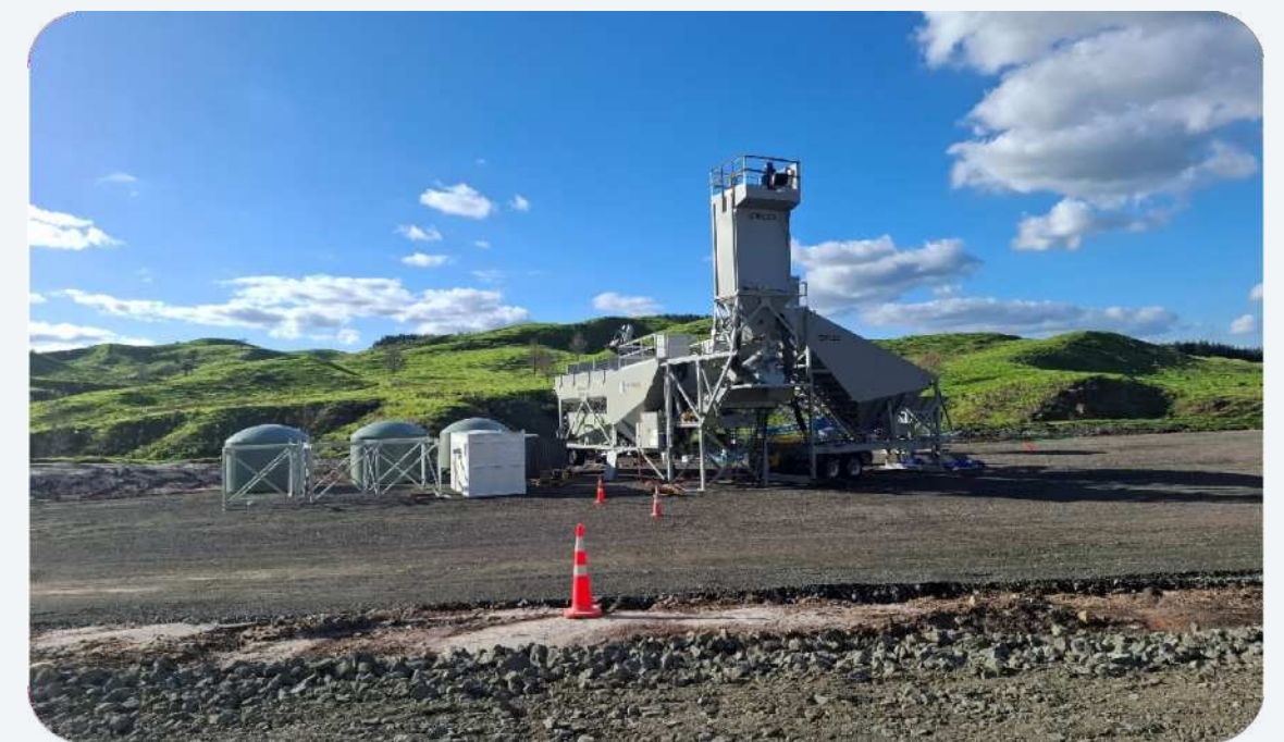
BATCHING PLANT INSTALLED FOR FOUNDATION POURS
