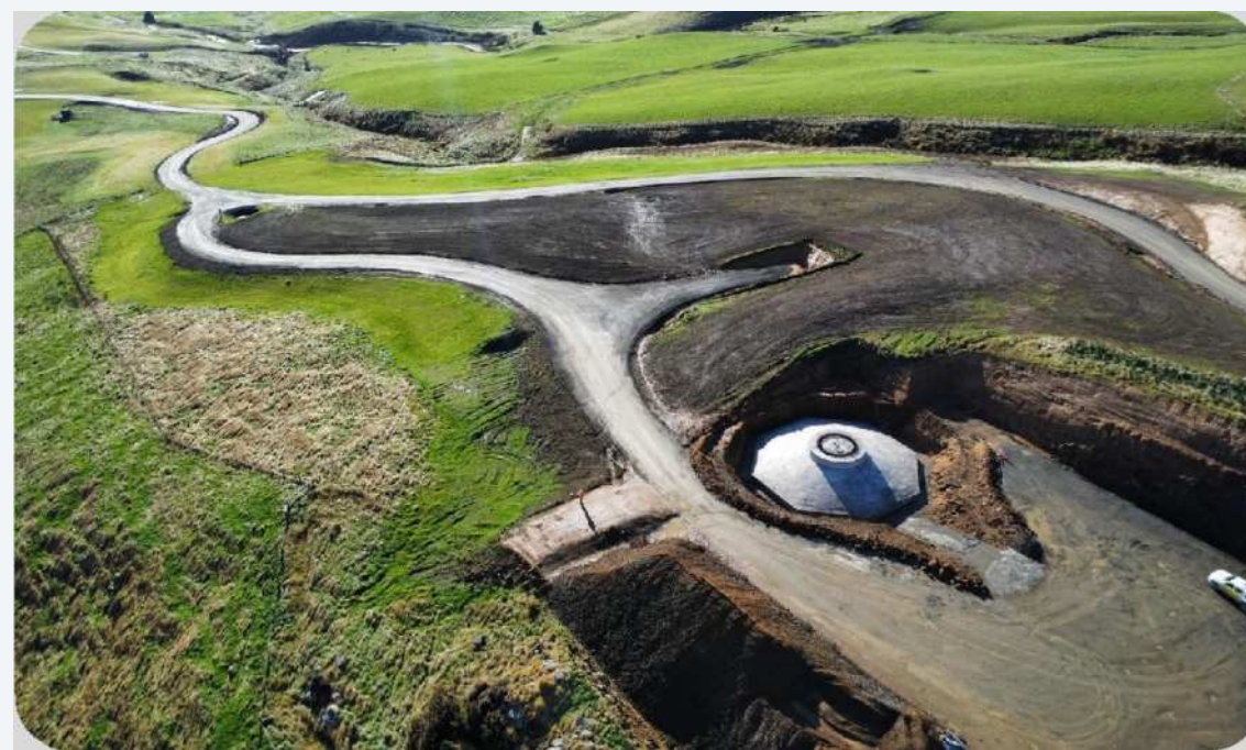
FINISHED ROADING, HARDSTAND & FOUNDATION
