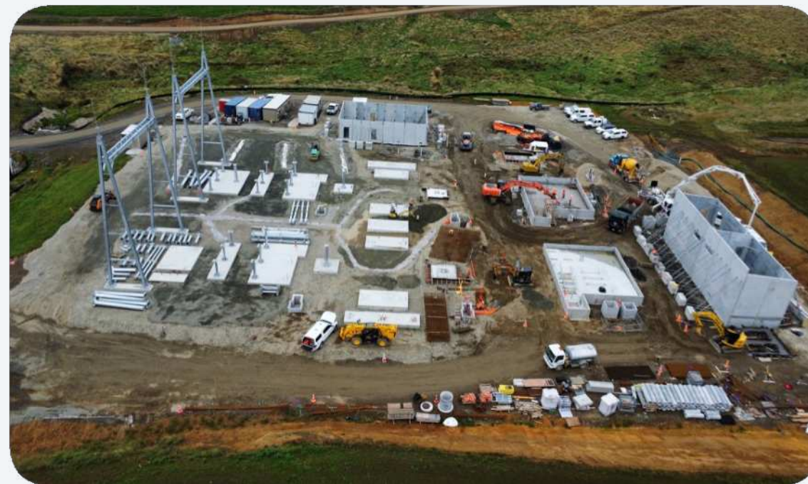
220KV SUBSTATION CIVIL & STRUCTURES ARE COMPLETE
