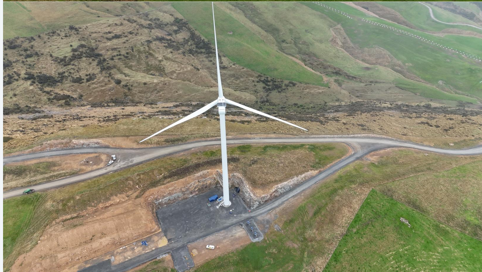
Kaiwera Downs Stage 2 under construction
