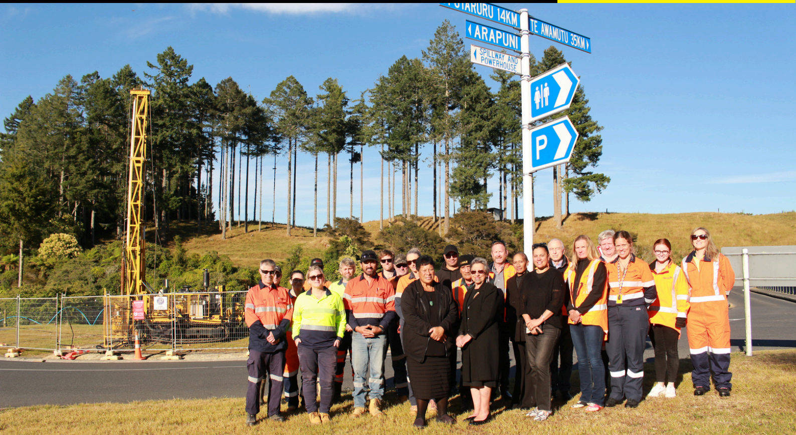
Ngaati Koroki Kahukura from Pohara Marae and Maungatautari Marae, with the project team, marking the start of drilling work on the left abutment at the Arapuni Hydro Dam in January 2025.
