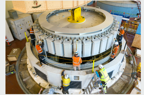
Precision work to install the rotor for Generator Two.
