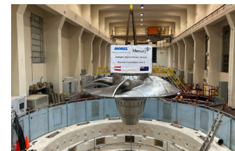
Lowering the turbine into the chamber.
