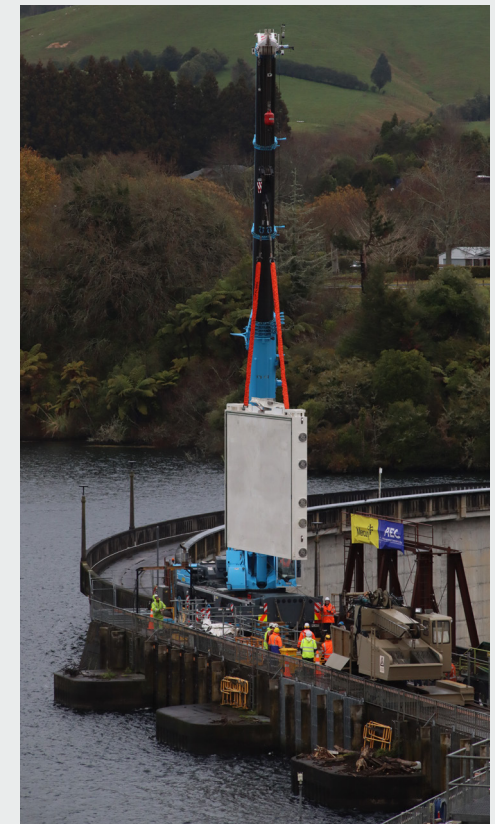
The gate being lowered into the hydro dam.
