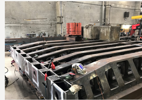
Fabrication of gate carcass at the AEC workshop.
