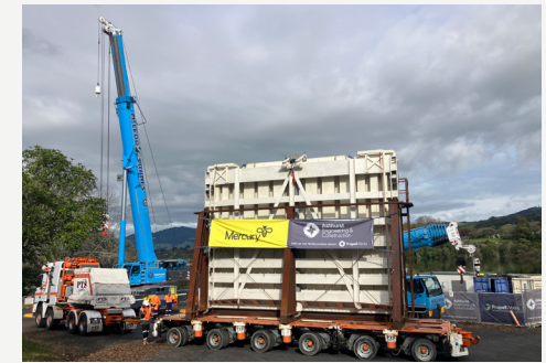
The gate is lifted into a cradle on a trailer and then reversed onto the hydro dam.
