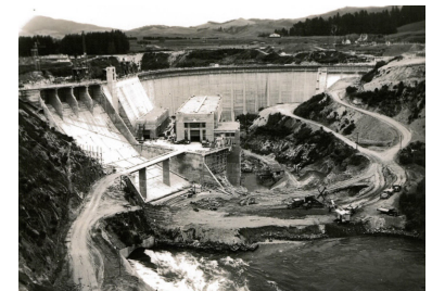
An aerial view showing the diversion tunnel, access bridge and dam completed.
